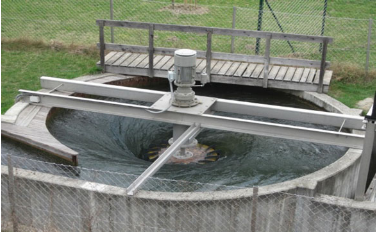
Fig. 1 Gravitational water vortex power plant [2]
